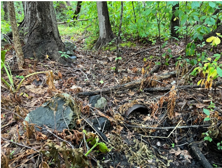
Photo taken August 23, 2022: View of clay pipe connecting wetlands.
