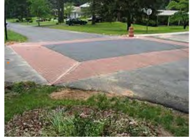
Raised Intersection at John St / Pleasant St
