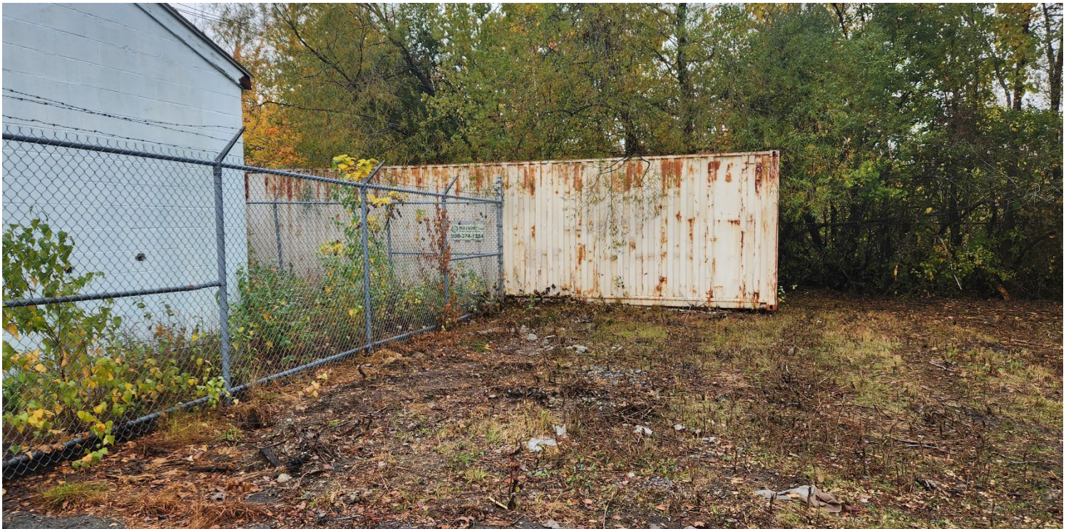
Photo #4: View of the rear of the pump building, showing the proposed location for the liquid storage tank. The area consists of a mixture of compacted gravel and broken asphalt surfaces. The internal security fence (pictured), will be expanded to encompass the tank. Facing northeast.
