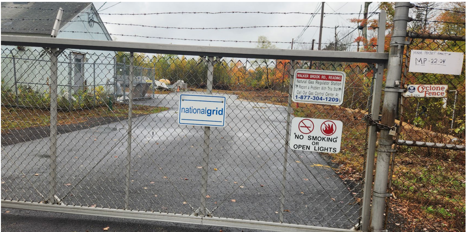
Photo #2: View of the site entrance, and exterior security fence. The existing building and current fence that will be adjusted for the tank installation can be seen on the left. Facing southwest.
