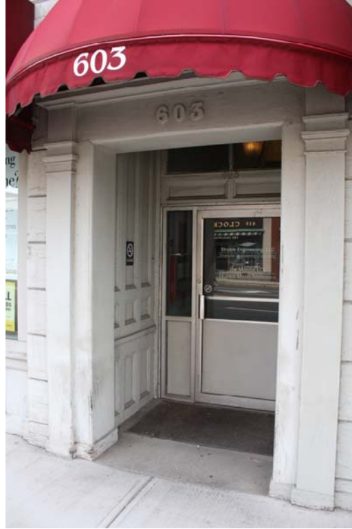
Entrance to upper level
