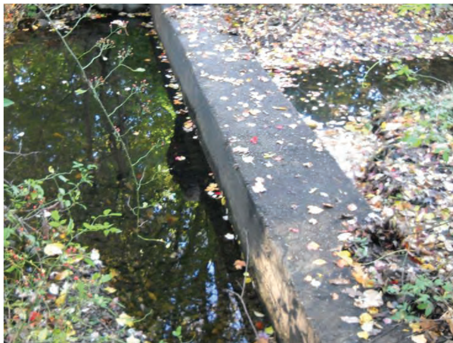
Figure 2-6. Pipe Encasement near Sunnyside Avenue
