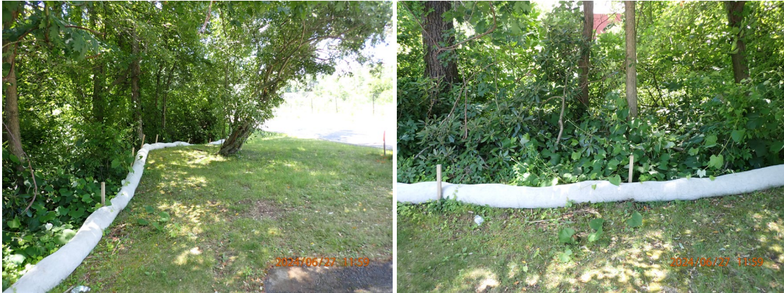
Construction Access Point
