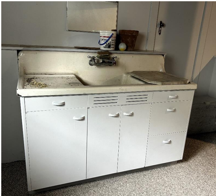
Original kitchen sink cabinet in laundry area.
