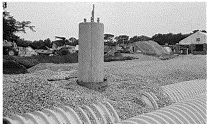
Figure 13 - Chamber bed placed around light post.
