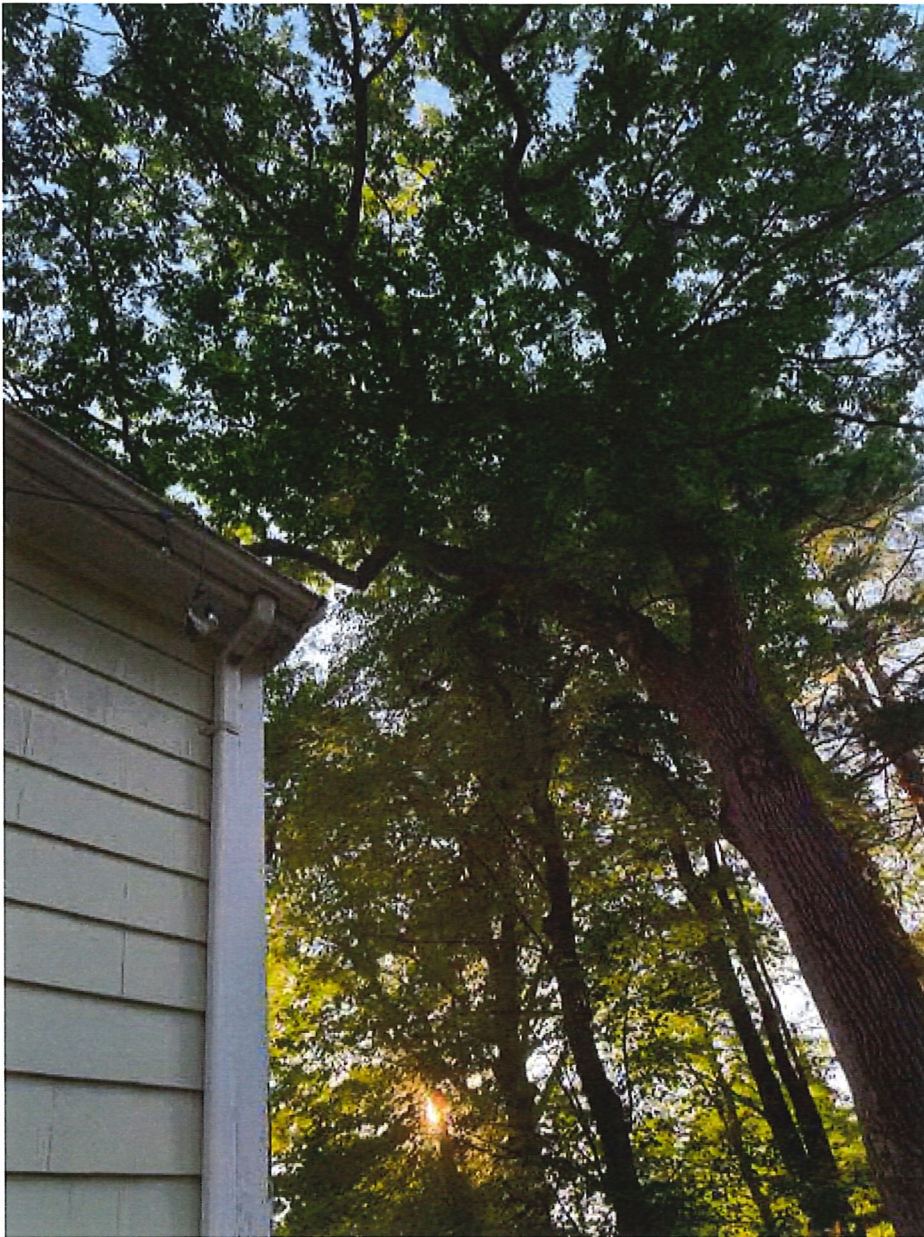
Trim to create clearance for roof and the structure
