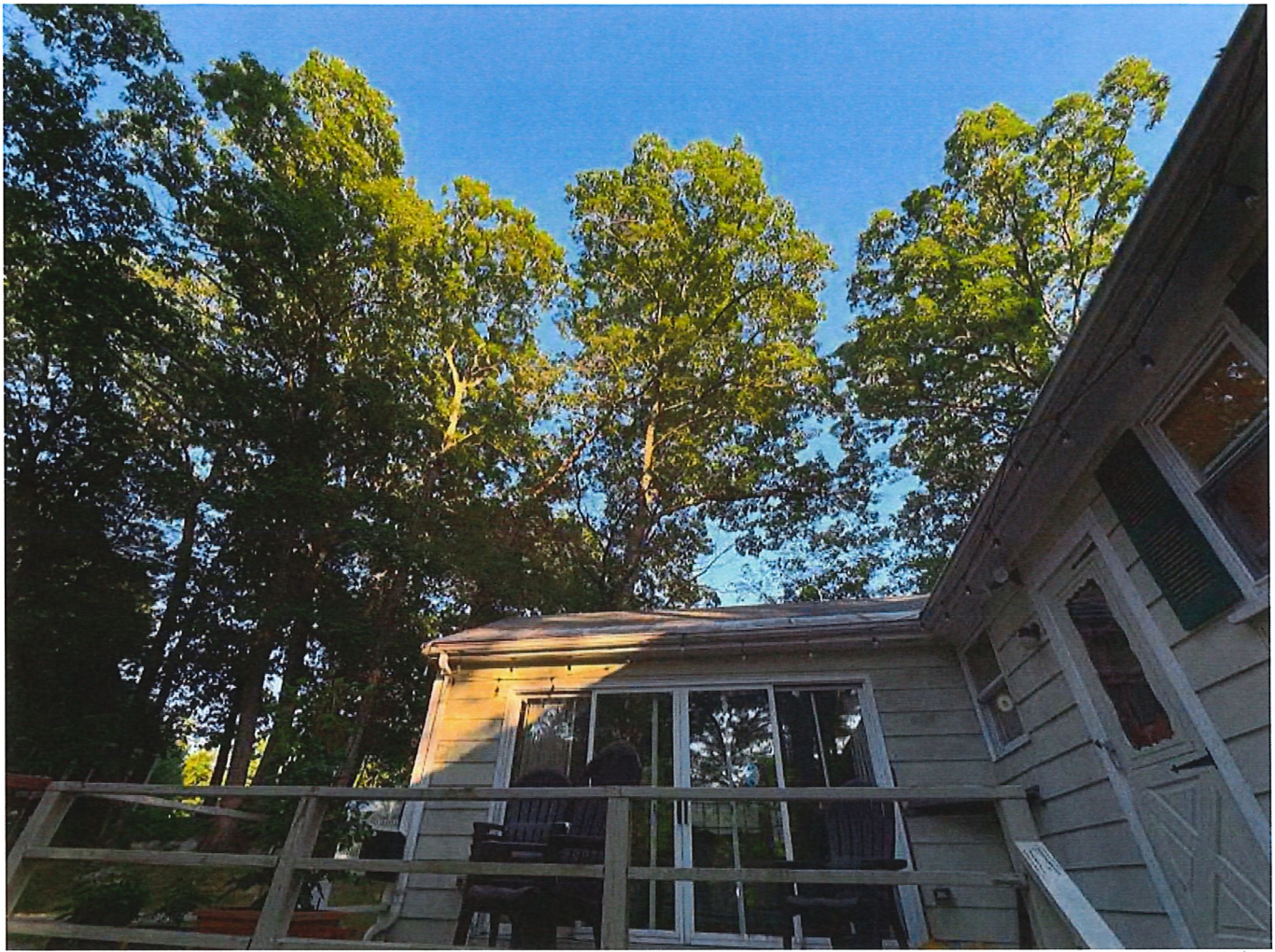
Trim to create clearance for roof and the structure
