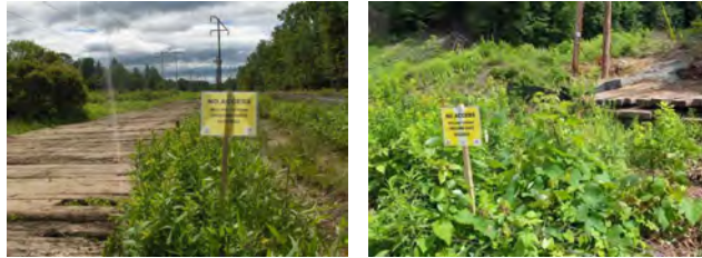
NO ACCESS – WETLAND/STREAM CROSSING MATS REQUIRED
