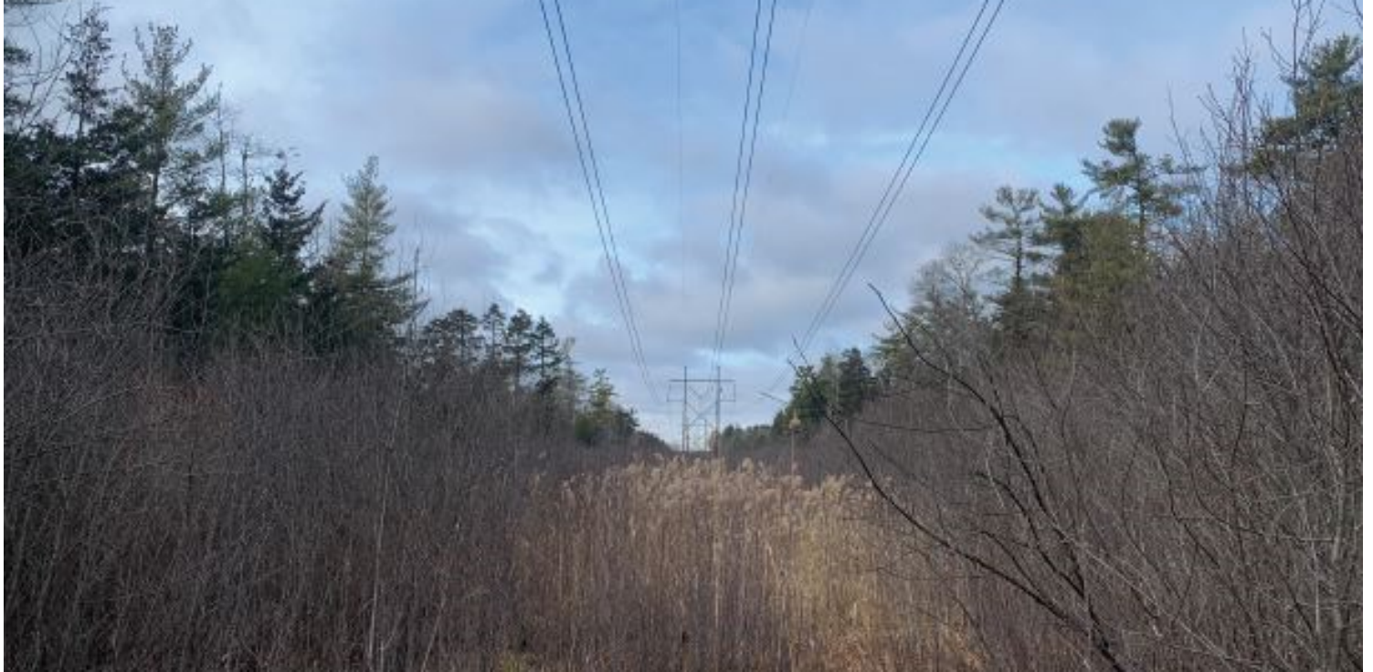
Photo #1: View of Structure 95, located within BVW. Activities within this wetland will include structure replacement and tree removals. Facing west.
