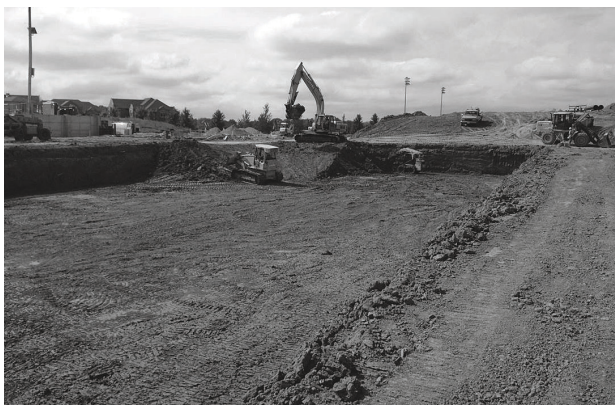
Excavate bed and prepare subgrade per engineer's plans.
