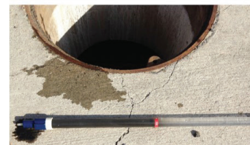
Inspection Utilizing Sediment Probe
