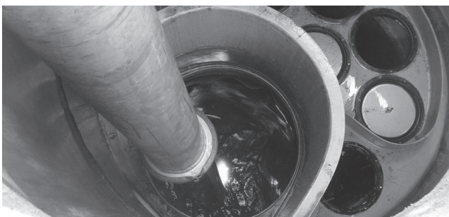
Vacuuming Sump Through MAW
