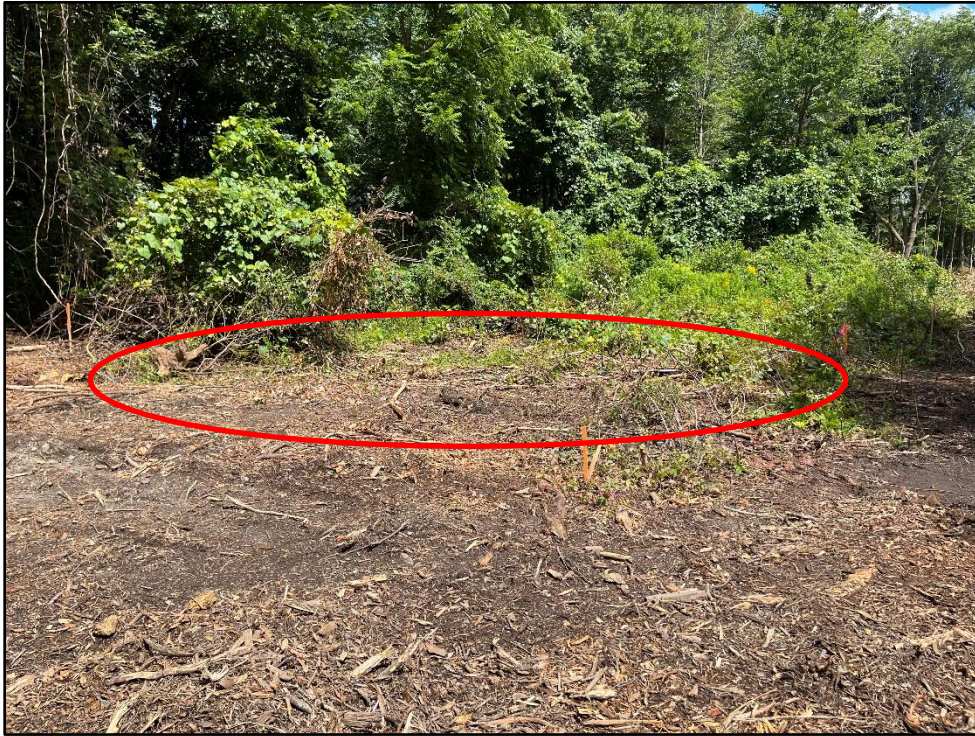
Photo 1. Wetland encroachment following tree removal and prior to ESC installation (Looking northeast)
