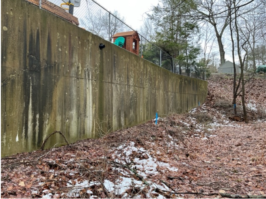
Retaining Wall – Looking South
