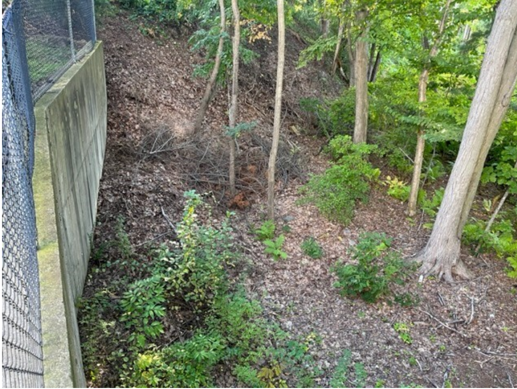
Retaining Wall and BVW – Looking South
